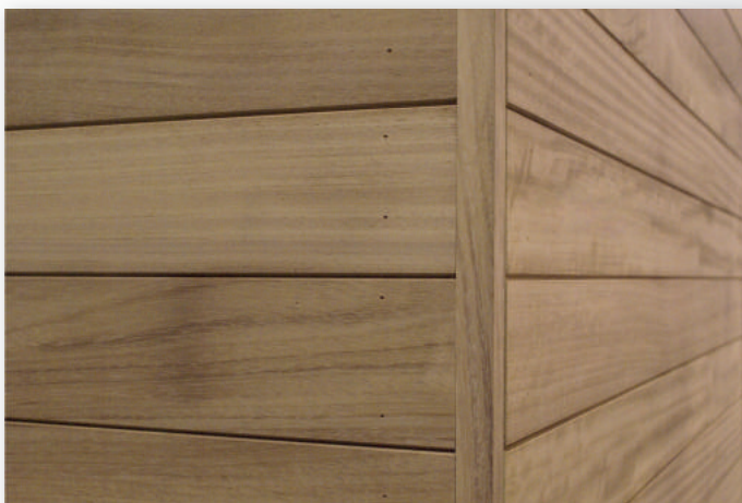
46 | DETAIL WAND & HOEK IROKOPROFIEL
