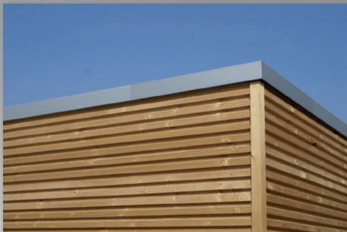
41 | DETAIL ALUMINIUM DAKTRIM
